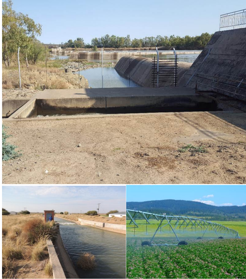
Figure 3. 4 Illustrations of Hartbeespoort WUA – Dam weir and outlets (top) and the main canal and center pivot irrigation system for cultivation (bottom).
