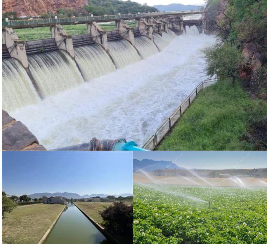
Figure 3. 5 Illustrations of Orange-Vaal WUA – Dam weir and outlets (top) and the main canal and sprinkler irrigation system for cultivation (bottom).
