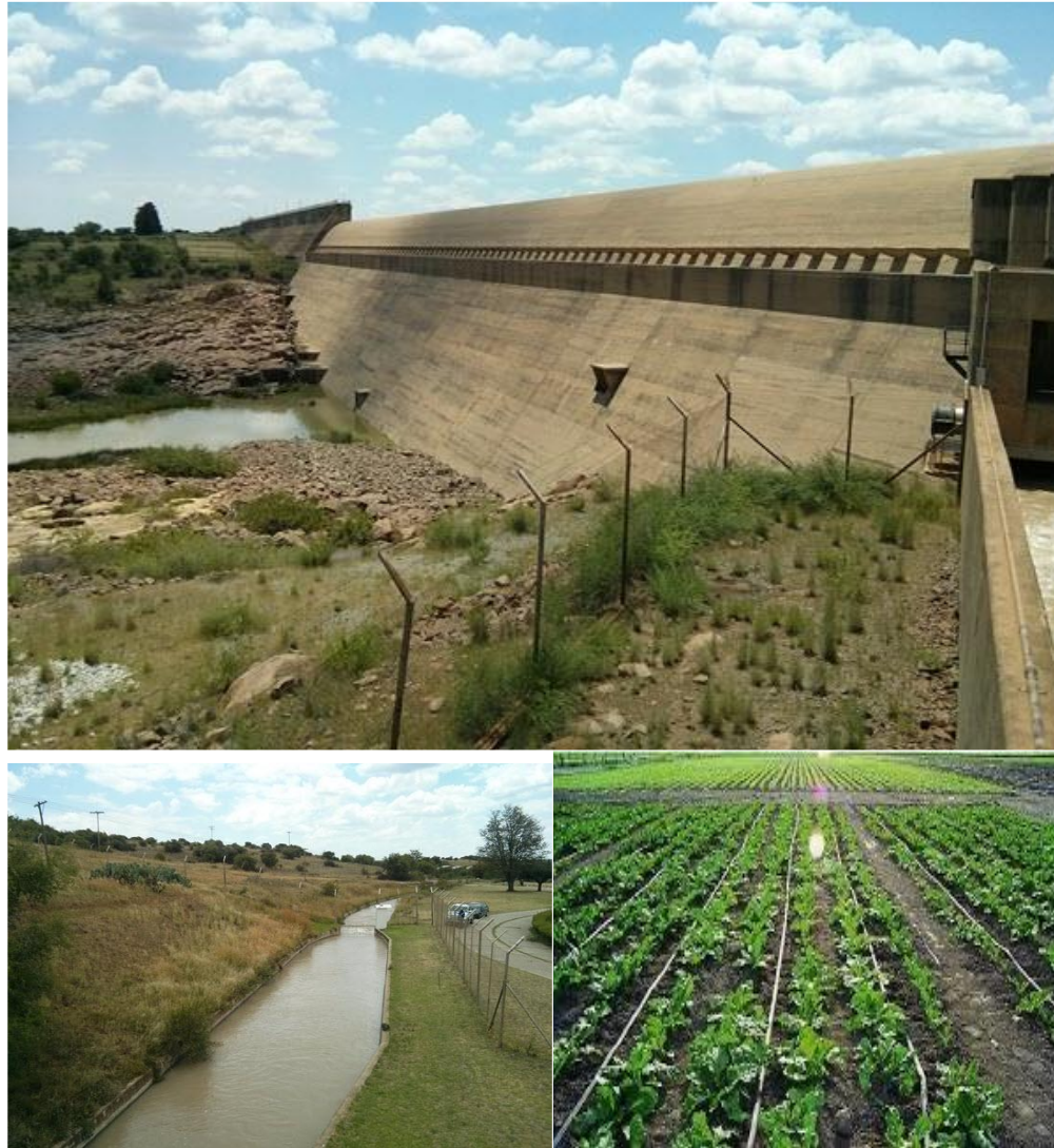
Figure 3. 3 Illustrations of Sand-Vet WUA – Erefenis Dam structure (top) and examples of the Vet canal system and drip irrigation for cultivation (bottom).
